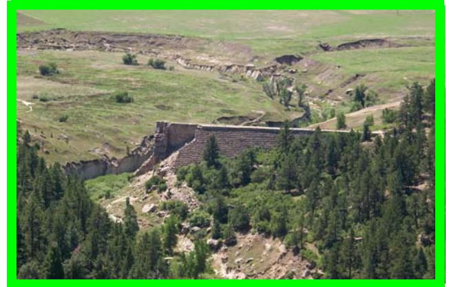
View of the Dam that burst in the 1965 flood
