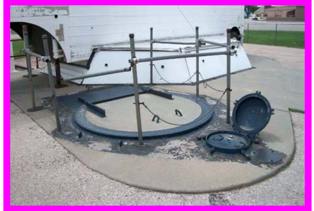
Maintenance access to the Silos is via a hatchway and a 30 foot vertical ladder. The Missile is actually launched remotely.
