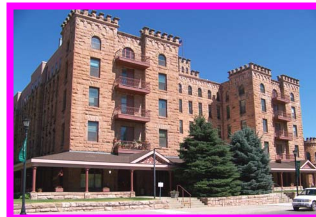
The 1891 Evans Hotel was the 1st Sandstone Bldg.
