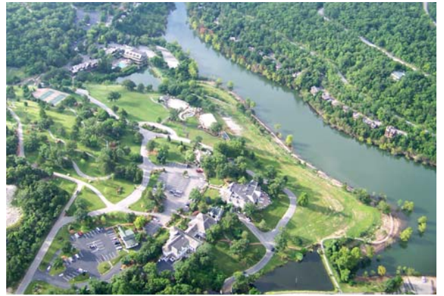
View of the Big Cedar Lodge resort complex
