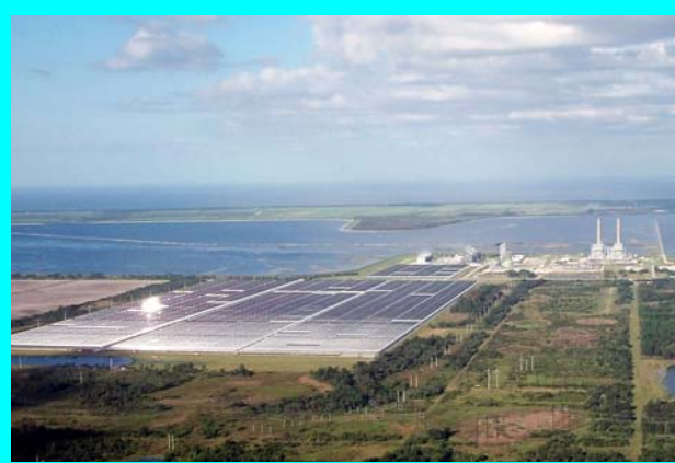
Martin Power Plant's 500 acres of solar panels
