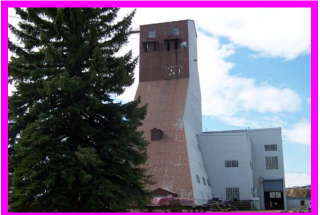
The mine's 5,000 foot vertical shaft elevator house
